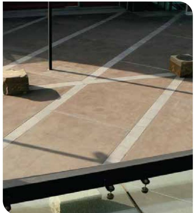
Project completed using CCS Obsidian
