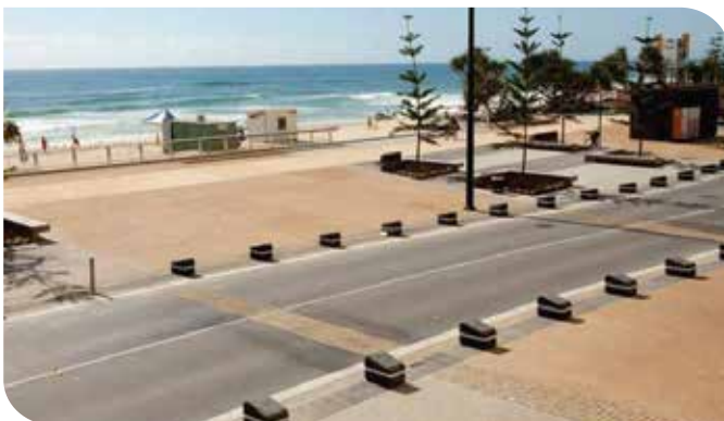
Pathway completed with CCS Kalgoorlie
